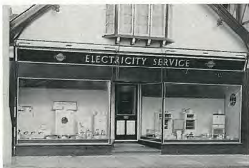
The present Service Centre in the Market Place at Winsford.
